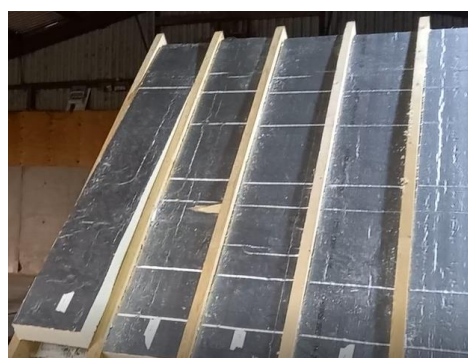
Placing the last board
