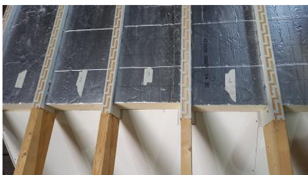
Track and insulation boards fitted
