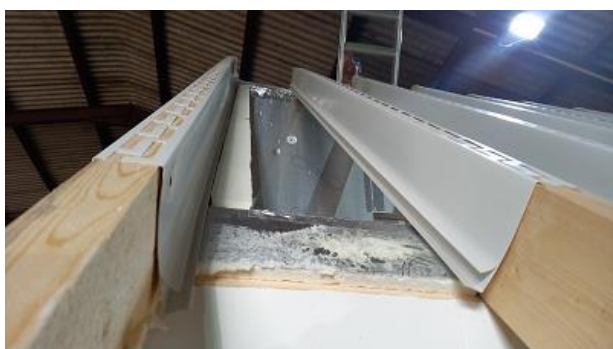
Installing the last few pieces of Insulfix Track
